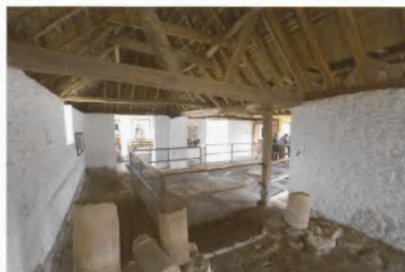
5 Interior view of one of the cover buildings over the north range at Bignor Roman villa, West Sussex. On the left of the picture Roman masonry is seen utilised as the footing for the cover building wall.
