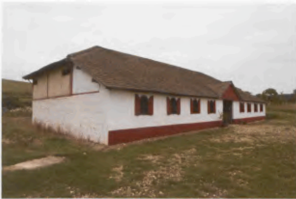
19 The reconstructed villa-house at Butser Iron Age Farm, Hampshire showing the roof design that resulted from compromises adopted to meet modern planning constraints.
