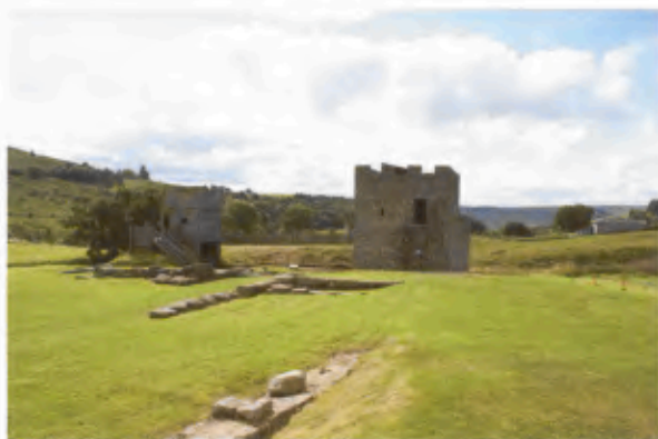
9 The ex situ reconstruction of a length of stone wall and a turret and a length of turf wall and a timber Milecastle gateway from Hadrian's Wall at Vindolanda, Northumberland.
